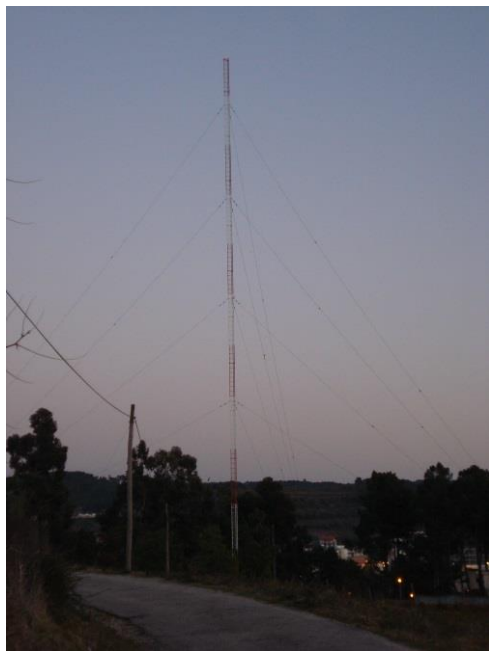
Vila Real MW transmitter for Rádio Sim - 981 kHz 1 kW (taken in 2008)
